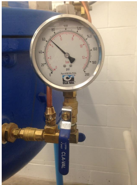
This UV system was currently processing 1870 Gal/Min and was operating just over 60 psi.
