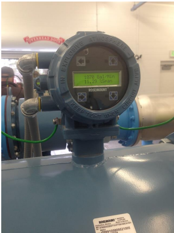
This UV system was currently processing 1870 Gal/Min and was operating just over 60 psi.
