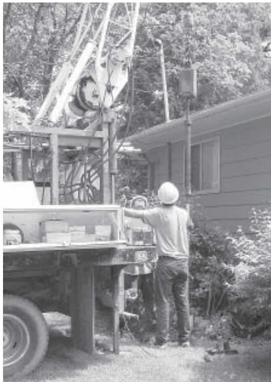
▲ A local well driller closes an abandoned well located in Lansing Township.
